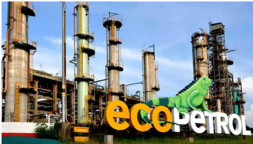
Ecopetrol Foto: Ecopetrol
