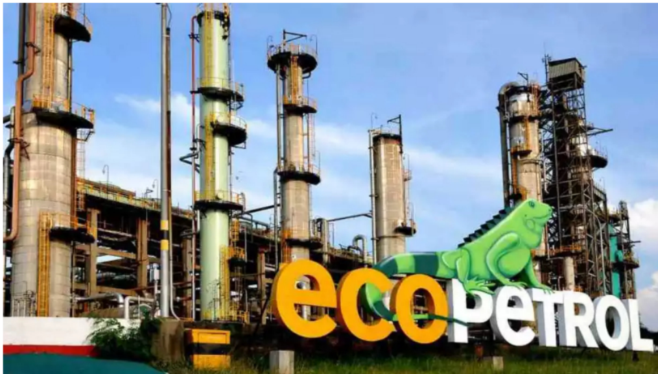
Ecopetrol Foto: Ecopetrol
