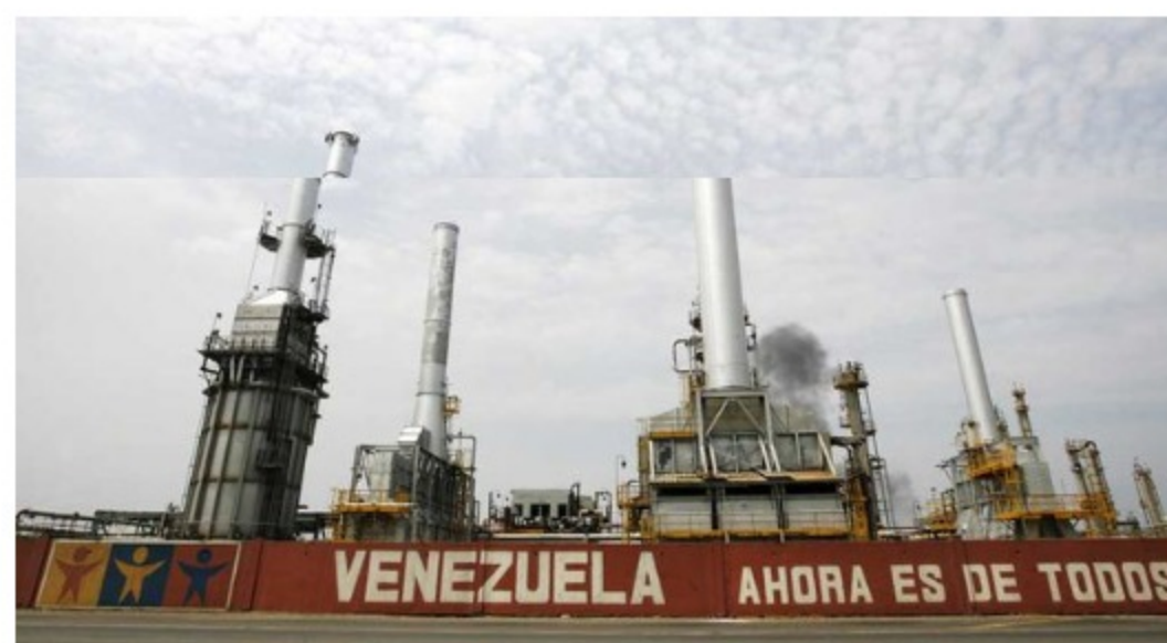
PDVSA's El Palito refinery is seen in Puerto Cabello, 150 miles (241 km) west of Caracas, September 23, 2009. Venezuela's state oil company PDVSA is still choosing partners for its Junin 10 oil field, a top PDVSA official said on Wednesday, contradicting his previous statement that France's Total was awarded the project. The banner reads: "Venezuela now belongs to all". REUTERS/Edwin Montilva (VENEZUELA ENERGY BUSINESS)
